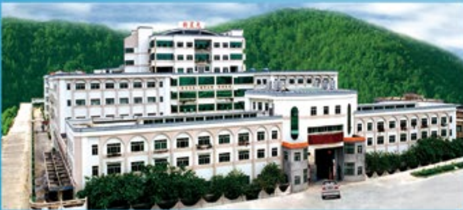
Our 90,000m 2 facility
